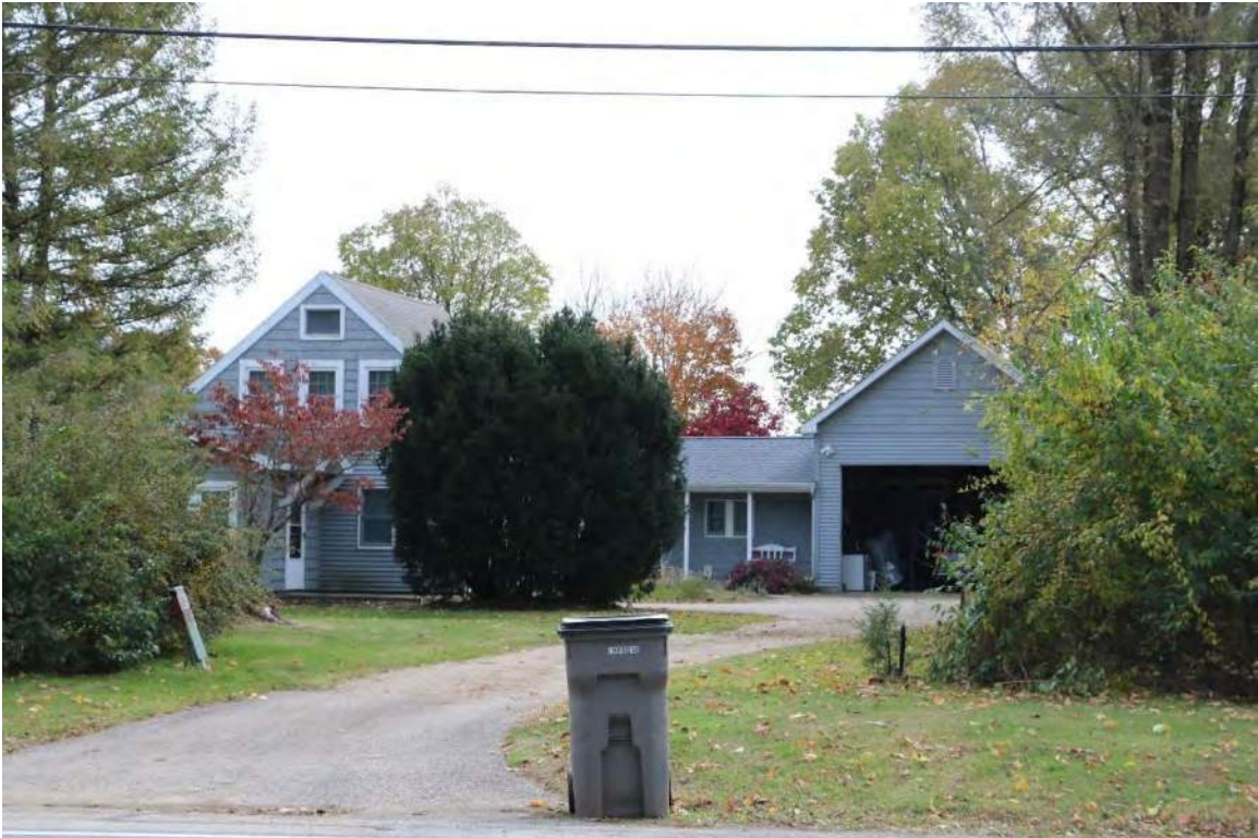
Photo 5. 2288 Yankee Street, view facing south.
