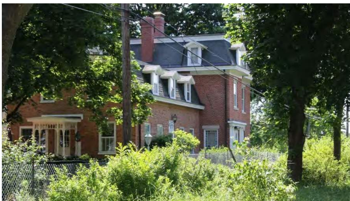
Figure 3. Side (east) elevation and north-facing facade, view facing west/southwest.
