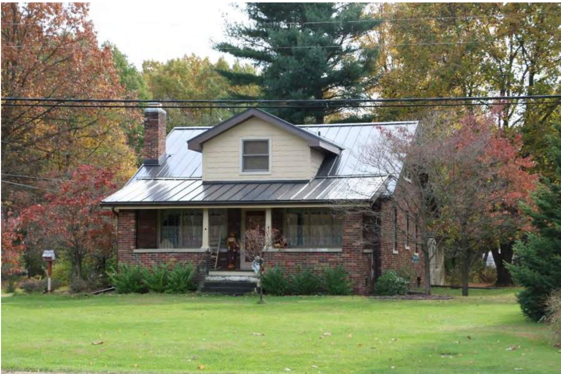
Photo 10. 2310 Yankee Street, view facing south.
