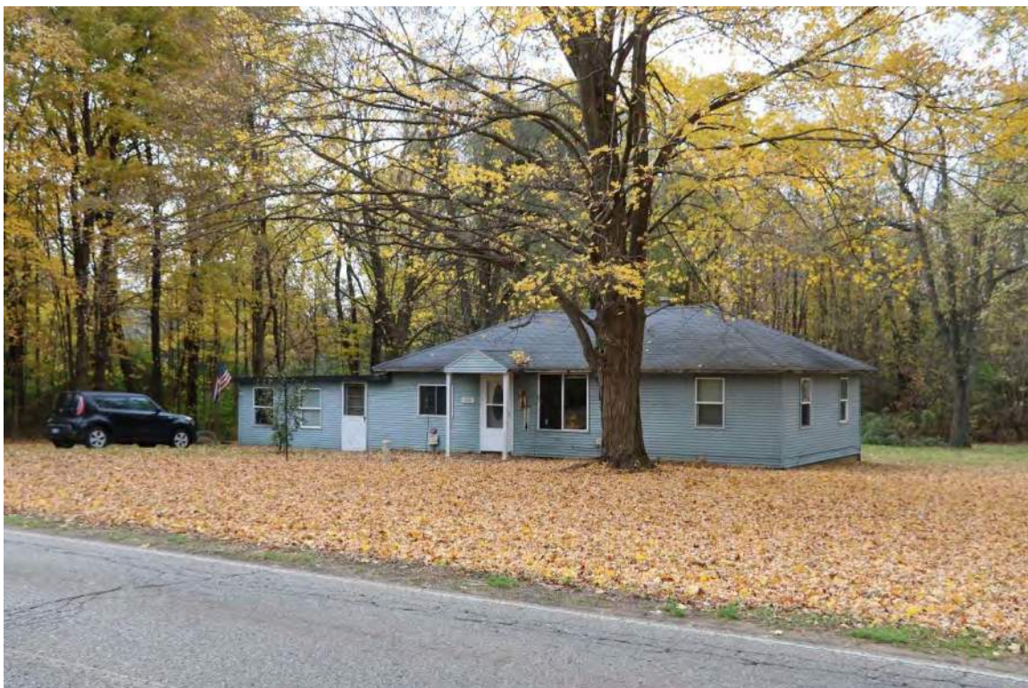
Photo 2. 1008 Carberry Road, view facing southwest.
