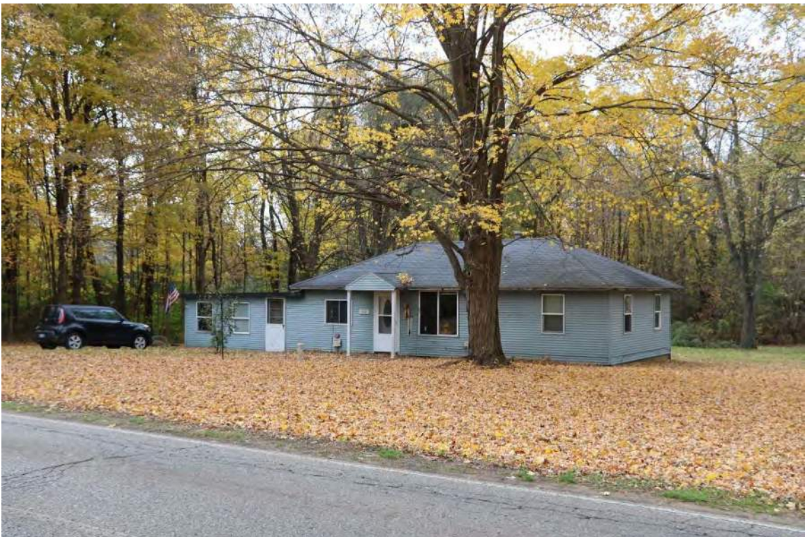
Photo 2. 1008 Carberry Road, view facing southwest.
