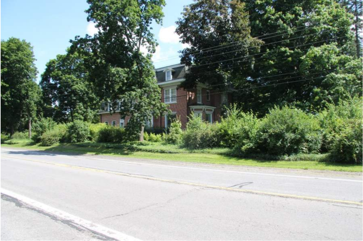
Photo A: View southeast from Yankee Street.
