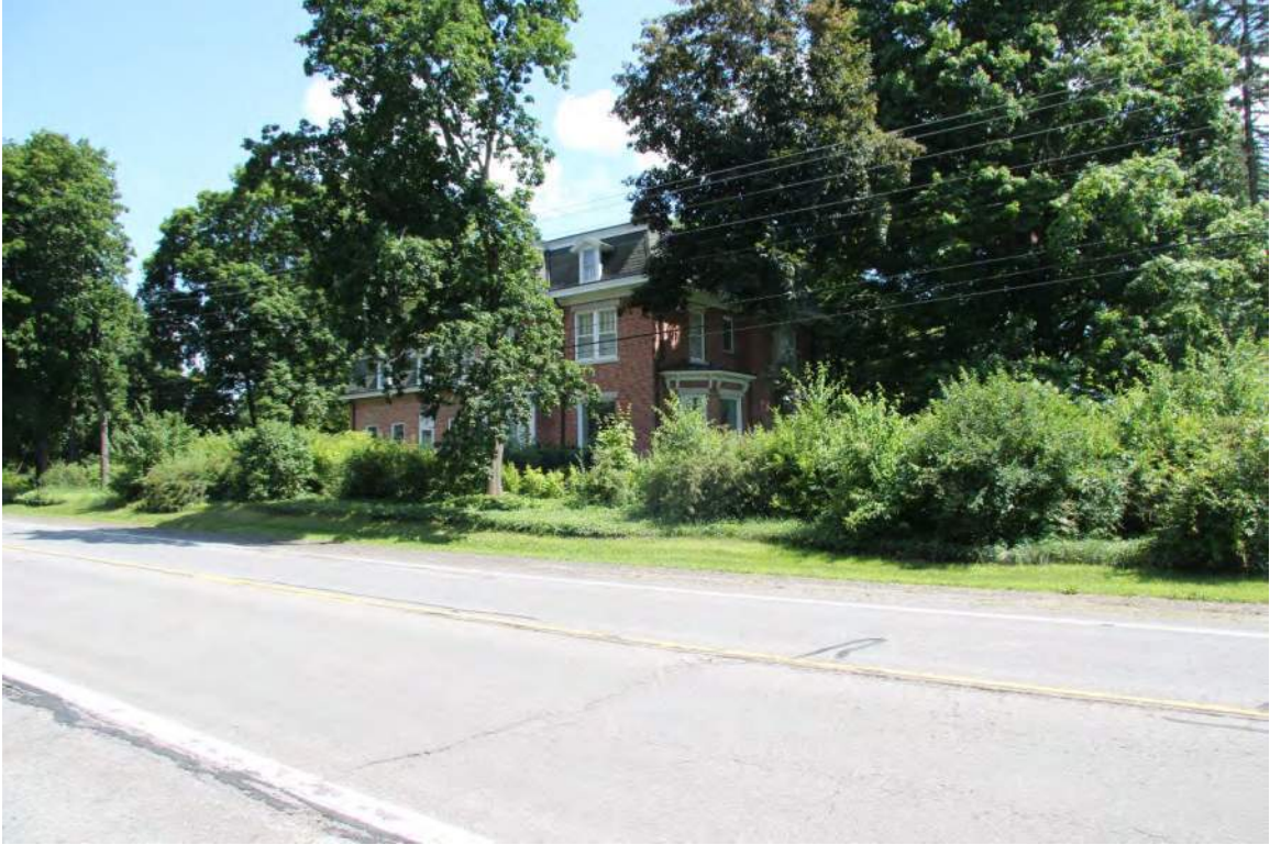
Photo A: View southeast from Yankee Street.
