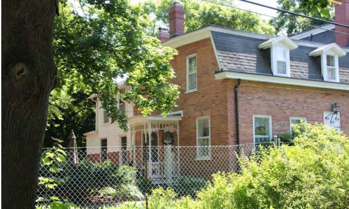
Figure 4. Side (east) elevation and north-facing facade of the original c.1832 house, view facing southwest.
