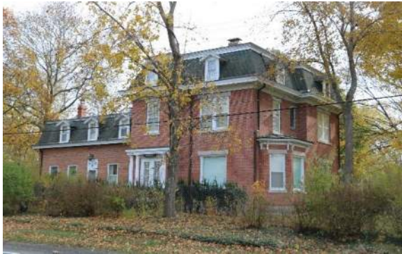
Figure 1: Pattengell-Milburn House at 2268 Yankee Street north (front) and west elevations, view southeast.
