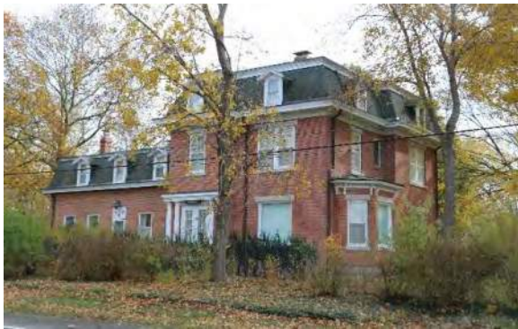
Figure 1: Pattengell-Milburn House at 2268 Yankee Street north (front) and west elevations, view southeast.
