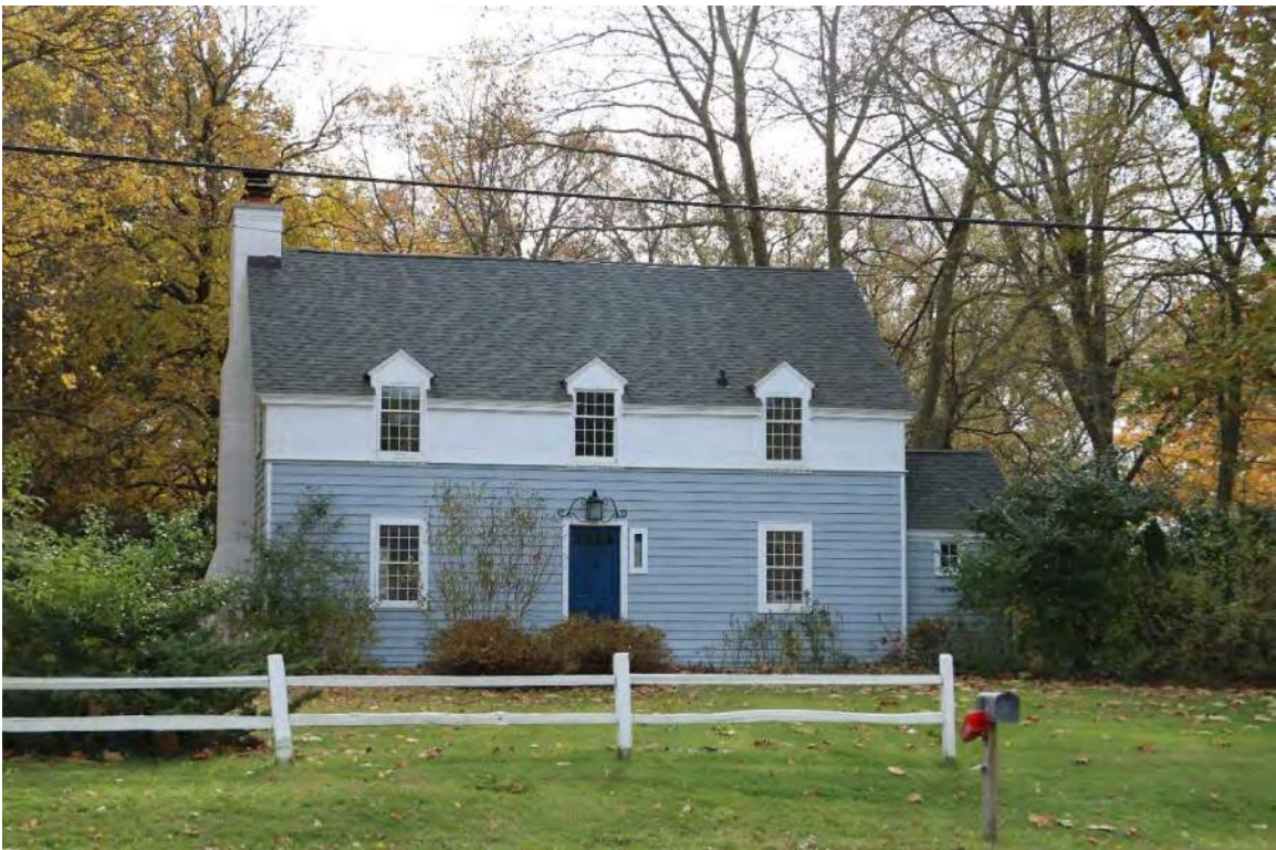
Photo 8. 2302 Yankee Street, view facing south.
