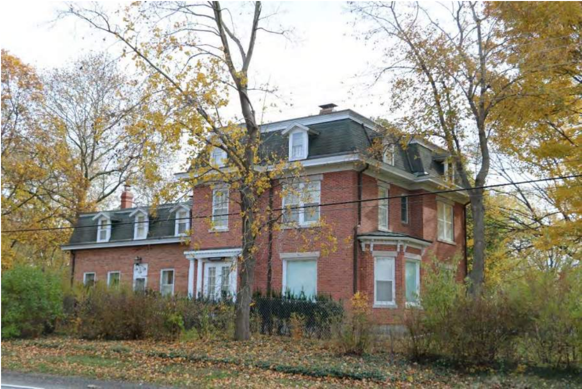
Photo 3. Pattengell-Milburn House, 2268 Yankee Street, view facing southeast.
