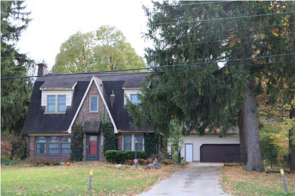
Photo 9. 2306 Yankee Street, view facing south.
