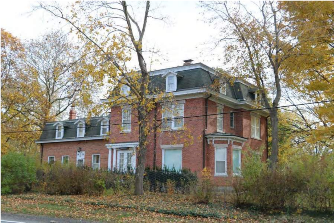
Photo 3. Pattengell-Milburn House, 2268 Yankee Street, view facing southeast.
