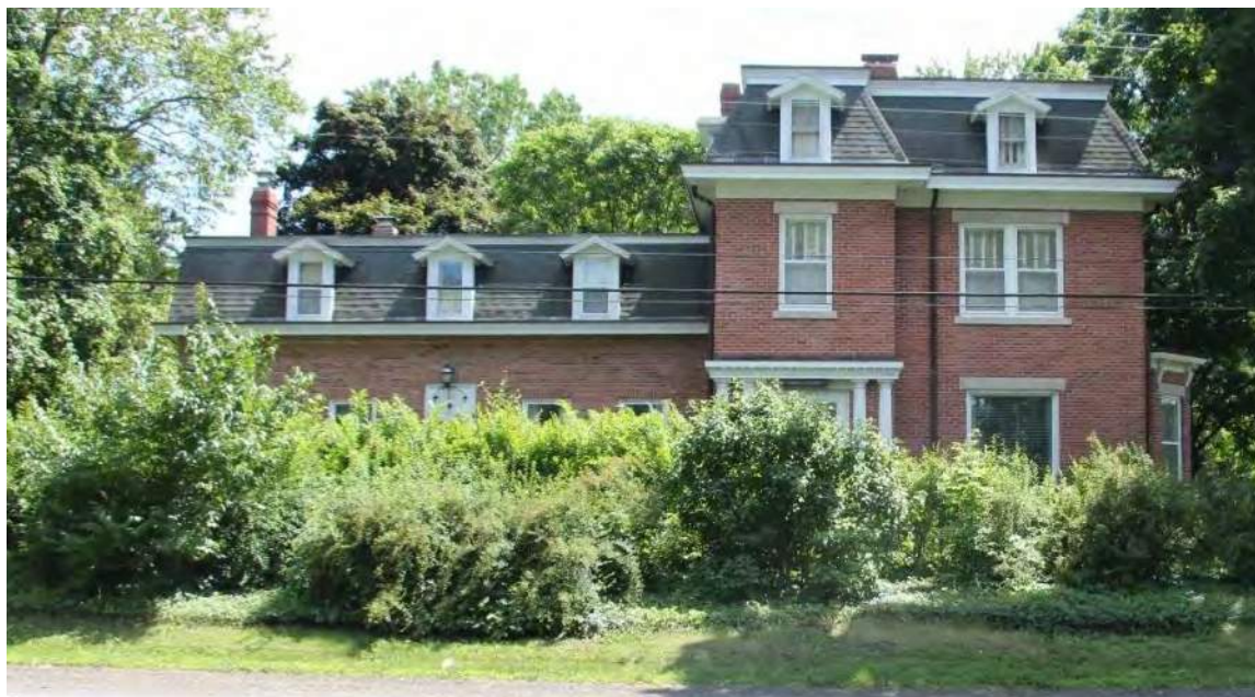
Figure 2. North-facing facade, view facing south. The original c.1832 house is at left and the c.1896 Second Empire-style addition is at right.
