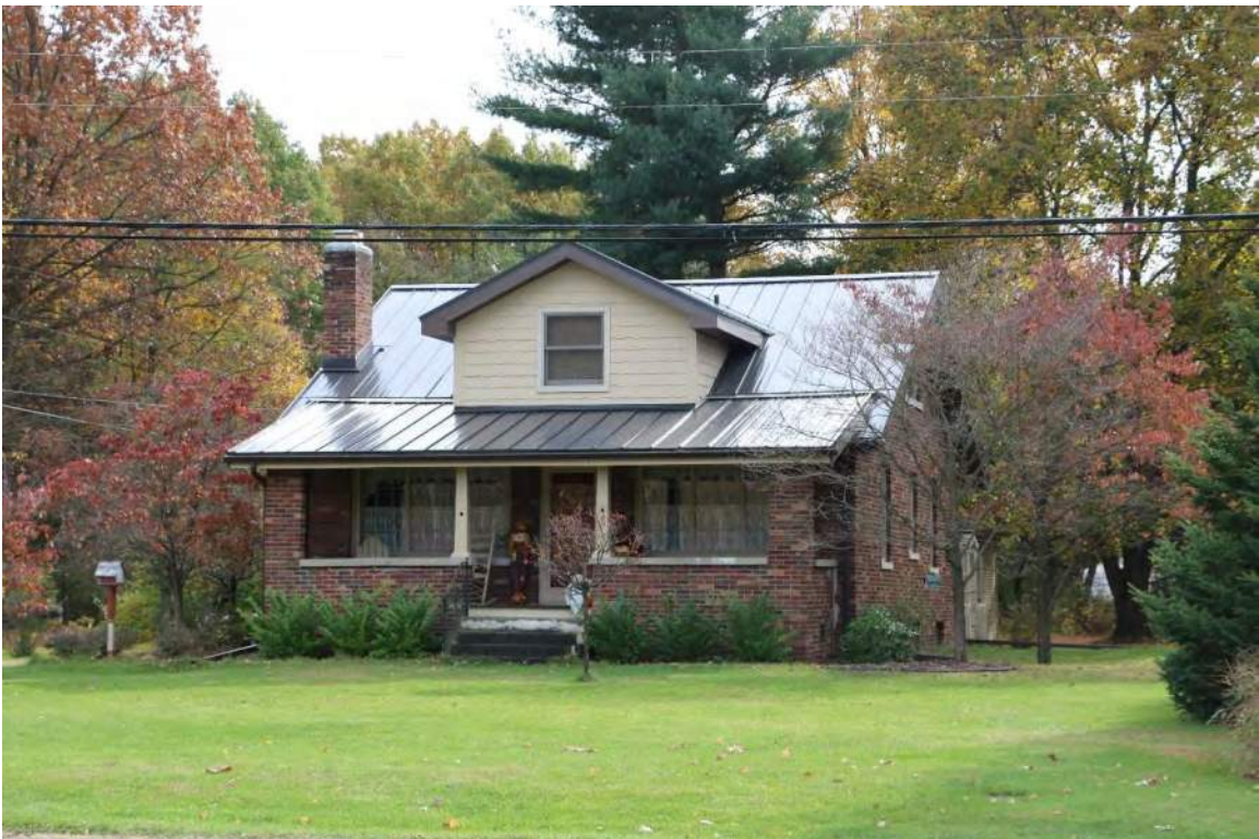
Photo 10. 2310 Yankee Street, view facing south.
