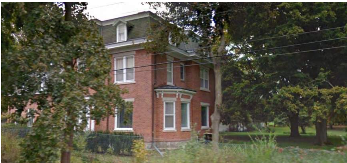
Figure 5. c.1896 addition, facing southeast, October 2018. Google Street View image.
