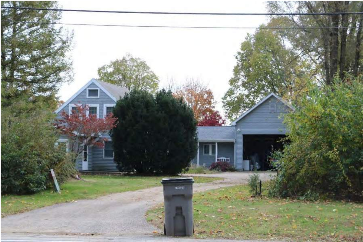
Photo 5. 2288 Yankee Street, view facing south.
