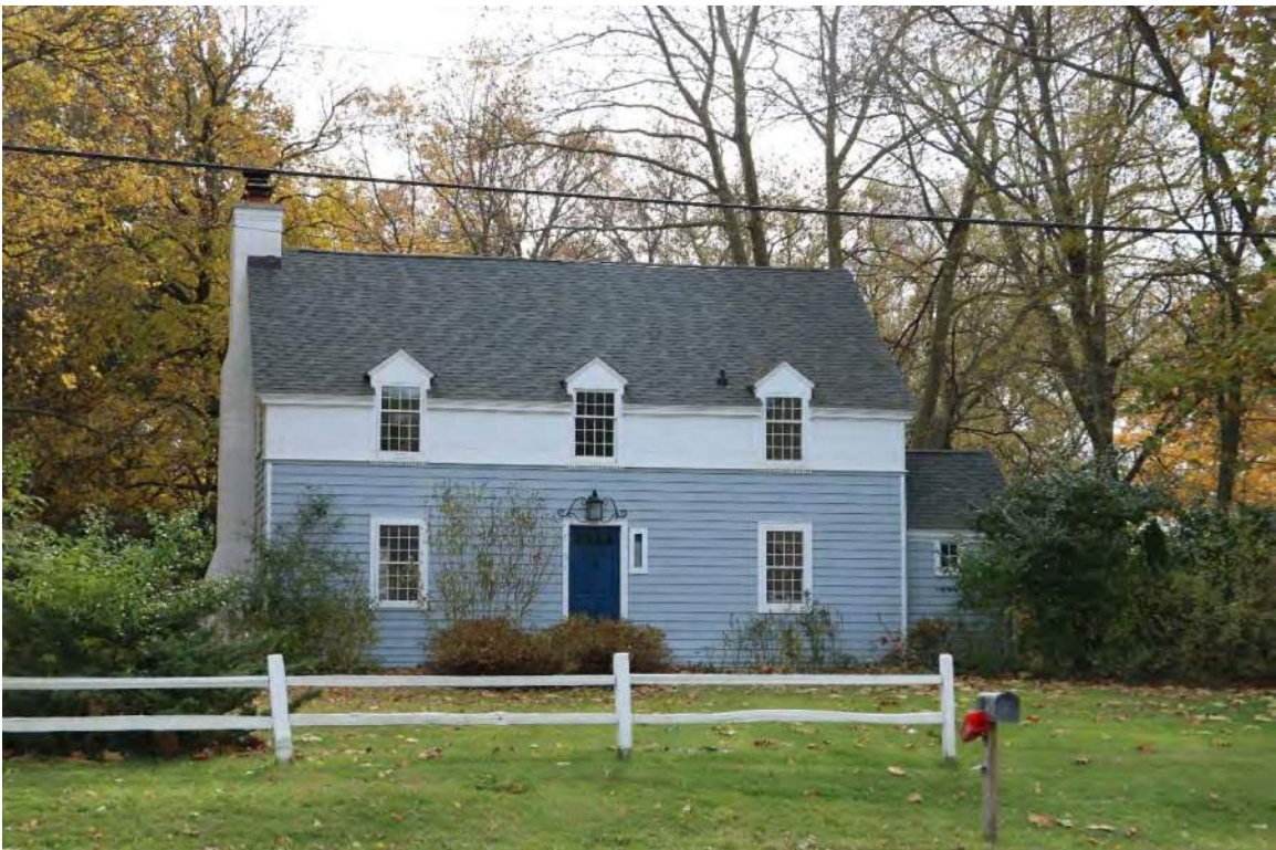
Photo 8. 2302 Yankee Street, view facing south.
